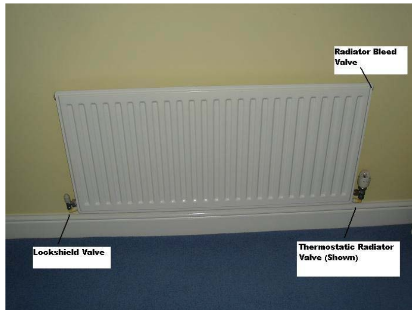
Figure 1 radiator valves
