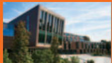
Emily Wilding Davison Building Our new state-of-the-art building, which opened in 2017, houses the library, Union shop, bank and exhibition space, as well as the Careers & Employability Service and other student services.
